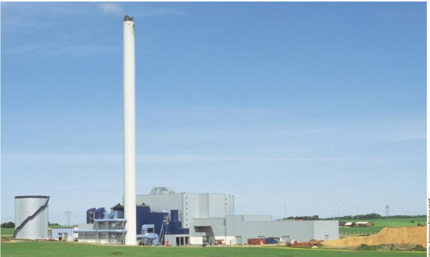
Maabjergværket (CHP plant). On the left, the storage tank of 5,000 m<sup>3</sup>. The straw storage is the low building on the right. Outermost on the right the outdoor wood chips storage.
