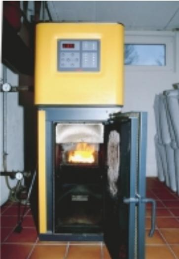
Today, several wood pellet-fired boilers have an efficiency exceeding 90 per cent and CO-emissions of approx. 0.002 per cent. Technically, this is about as good as it gets, unless the plants are fitted with flue gas condensation equipment.
