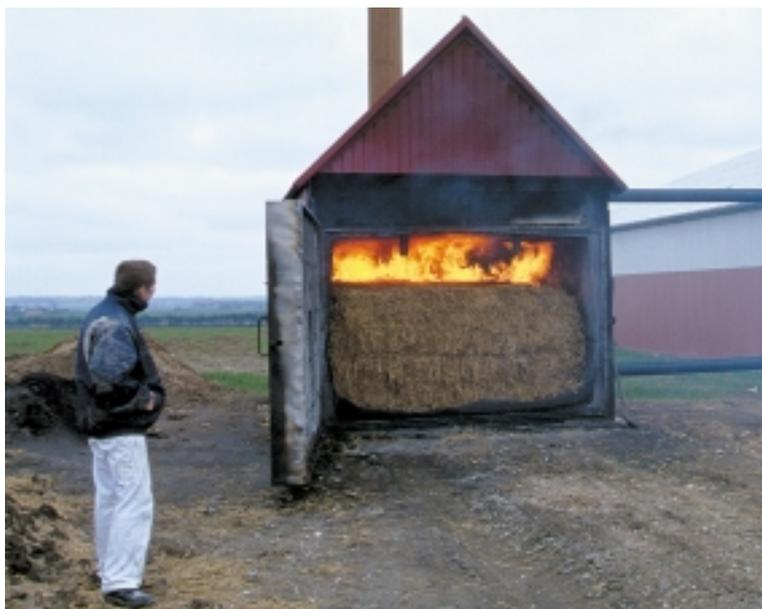
The efficiency of the manually fed straw-fired boilers has increased from 30-40 per cent in the 1970's to more than 80 per cent today. This means that manually fed plants are as efficient as automatic ones. On the other hand, the automatic plants generally require less service, and the carbon monoxide emission is lower. This favours the environment and reduces the amount of obnoxious smells, which is particularly important if the plant is located close to residential areas.
