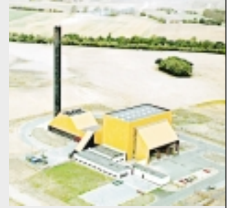
I/S FASAN Waste-to-Energy Plant
