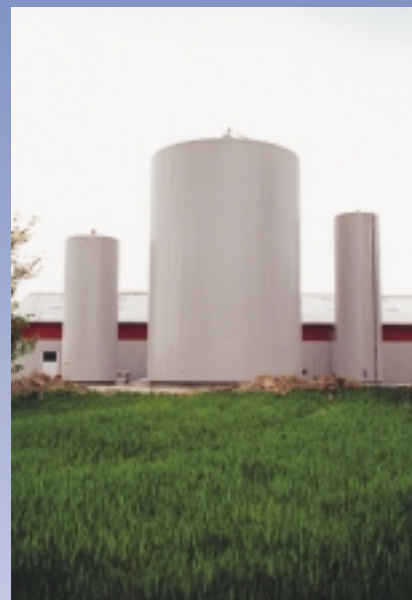
Smedemester farm biogas plant at Hadsund. The plant has a reactor of 600 m 3 and a 400 kW dual-fuel engine.
