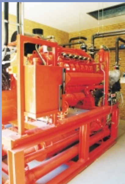
400 kW dual-fuel engine.
