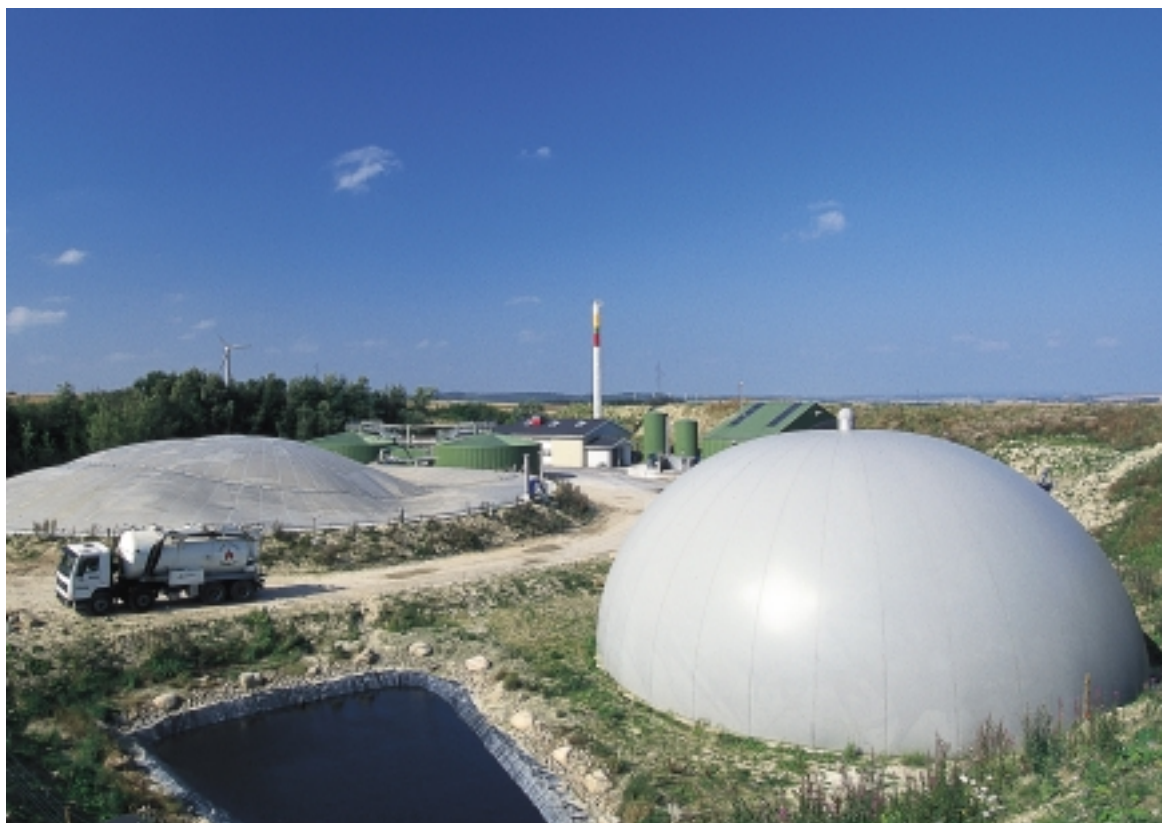
The centralised biogas plant at Vaarst-Fjellerad processes organic household waste from Aalborg in addition to livestock manure and industrial waste.
