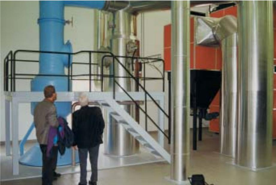
*Mist eliminator in brilliant blue and insulating jackets with glittering surfaces situated on the flue gas condenser. The boiler room at Græsted Varmeværk being demonstrated to a foreign visitor look like a "sitting room".*
